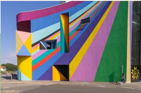
Towner Gallery, Eastbourne
